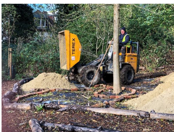
BWS placing sand in the Orchard
