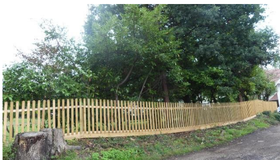
Fence along Hamilton Way
