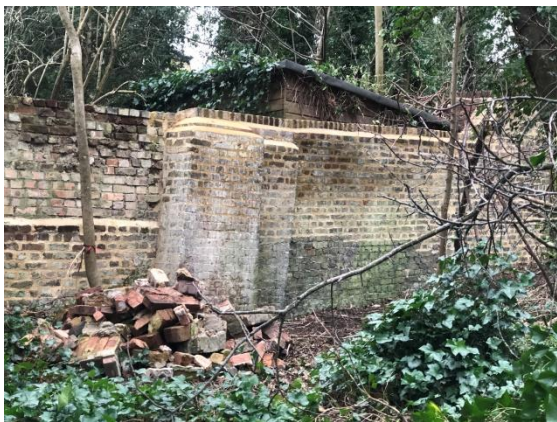
Part of the repaired wall
