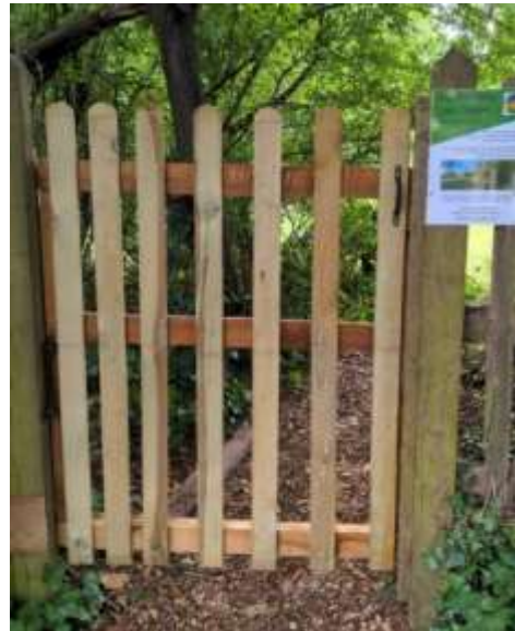
New gate in the unpaved section of Hamilton Way
