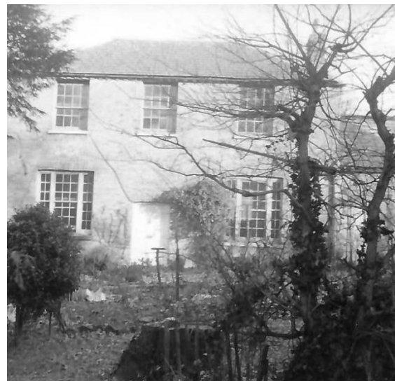
Photo showing an entrance to Brent Lodge
